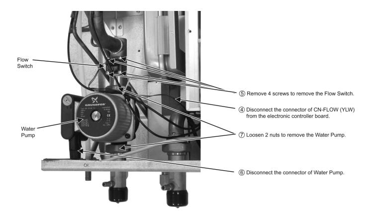
$\triangle$  When reinstall the water pipe, use grease or water at the joining.
