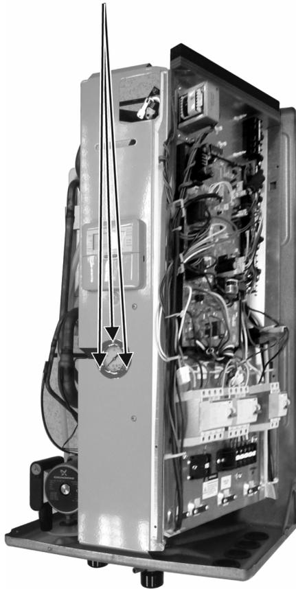
② Use spanner to release nut of pressure gauge.
